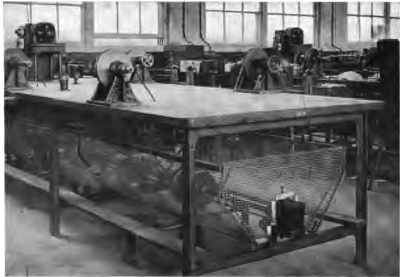
Fig. 2. Skirt Guards for Shafting. (Courtesy General Electric Co.)
